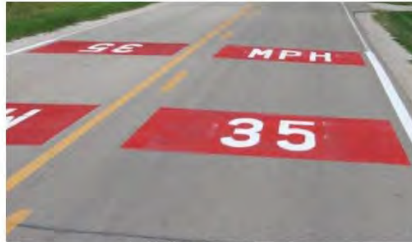
Pavement Speed Limit Markings
